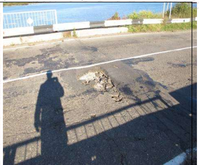
3-rasm. To'sin plitalari orqali suvningeerkin kirib borishi
